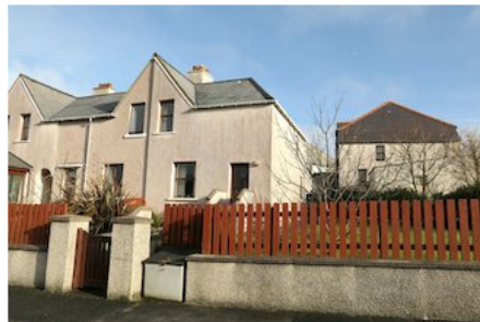
56 Haldane Burgess Crescent from front
