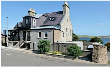
Rear of Leog House, showing entrances to flats.
