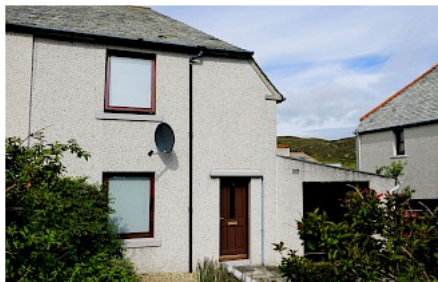
45 Haldane Burgess Crescent from front.
