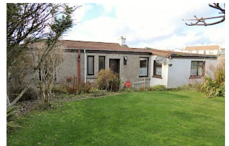
Rear of Beach Cottage
