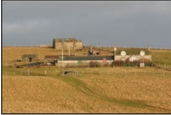
North Leadie with most of the outbuilding including Garages to the rear
