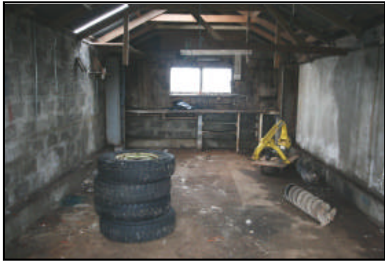
Inside of Garage
