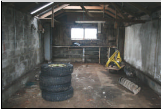
Inside of Garage
